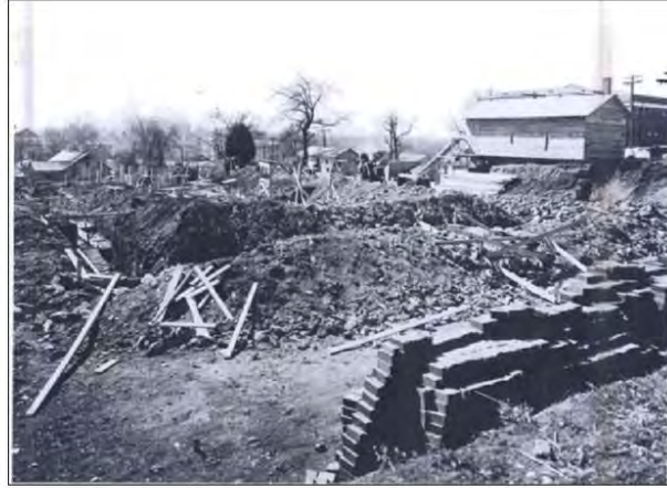
1938 construction of Baldwin Hall A Pictorial History of the University of Georgia, (Boney 2000)
